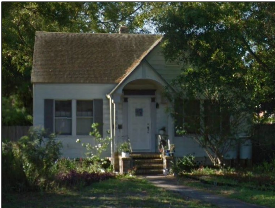
Figure 4: Primary residence at subject property, as shown in March 2015 Google Street View image, with composition shingle roofing
